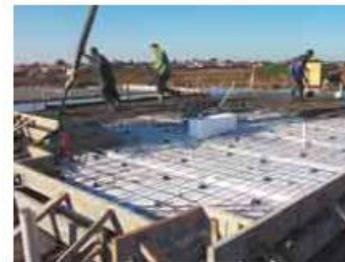
**Step 6** In a single concrete pour, partially cover the VoidForm® before filling the ribs. (This will help prevent the VoidForm® from floating).
