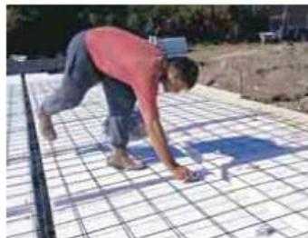
**Step 5** Place chairs under the mesh at a rate of 4 per VoidForm®.
