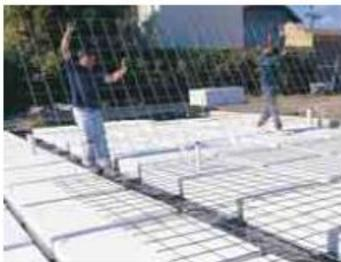
**Step 4** Place the reinforcement bars between the VoidForms® and the top mesh over the total area. Ensure tie laps are used as required.
