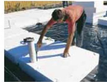
**Step 3** Starting from the corner of the site, lay VoidForms® in grid pattern, using Void-Lock® grid spacers. The VoidForms® can be easily cut to size and to fit plumbing fixtures.
