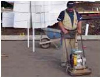
**Step 1** The building site must be levelled, all plumbing pipes fixed in place and the formwork positioned.
